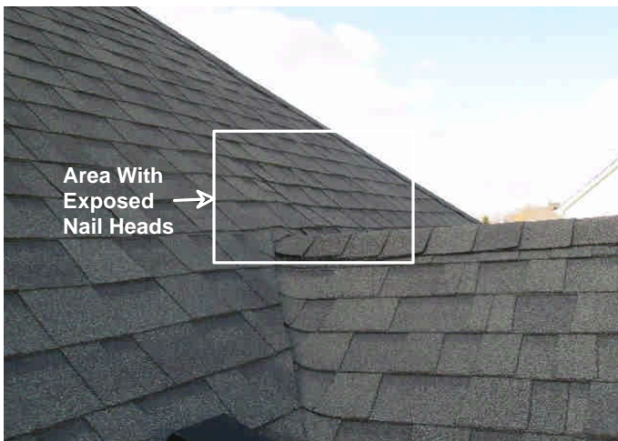
Figure Set - 1 Exposed nails heads
