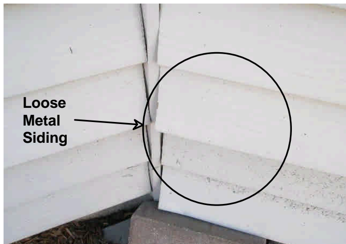
Figure Set - 6 Loose metal siding
