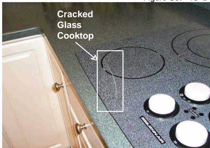
Figure Set - 14 Cooktop should be replaced
