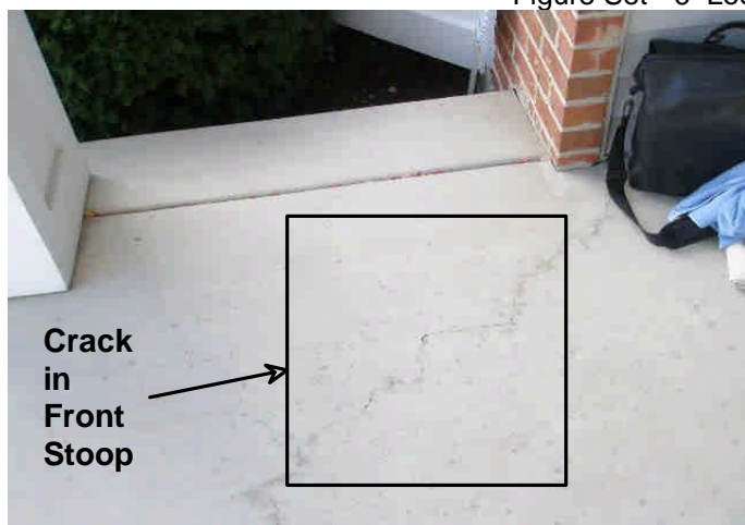
Figure Set - 7 Shrinkage cracks in concrete stoop
